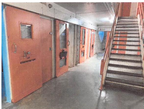
Prior to repainting
