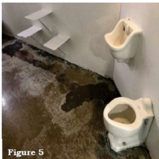
Figures 5 and 6. Leaking Detainee Cell Sink and Toilet, with Floor Mold in a Vacant Cell Located in an Occupied Housing Unit (left) and Housing Unit Ceiling Mold from Leaks (right)
