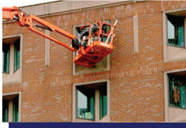
Window repairs at the Nashua Street Jail
