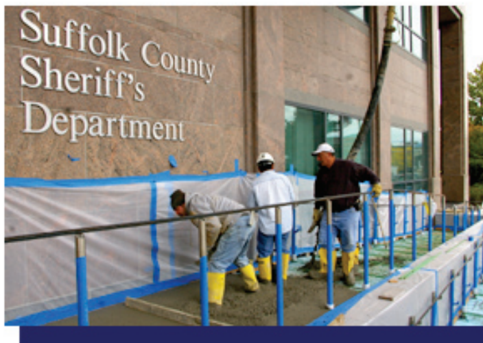
New construction in front of the Nashua Street Jail
