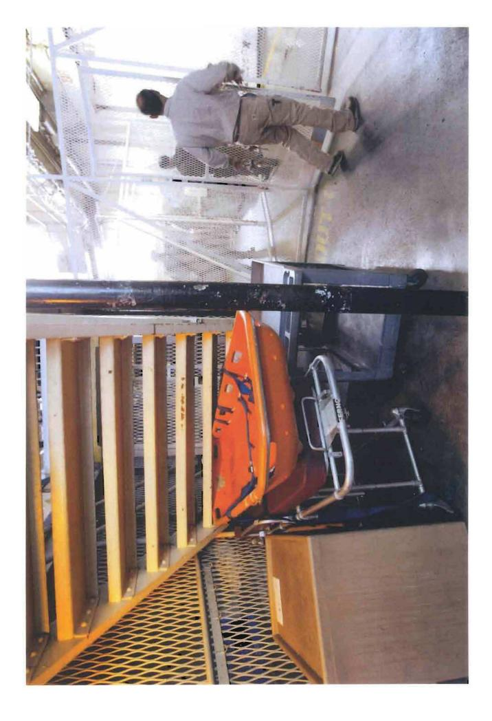
**1B:** The second tier inmate shower is visible (orange interior) directly over a mildewed shower curtain hung to protect medical and custody staff and patients from the streams of water that flow over the railing and onto the floor when the shower is in use.
